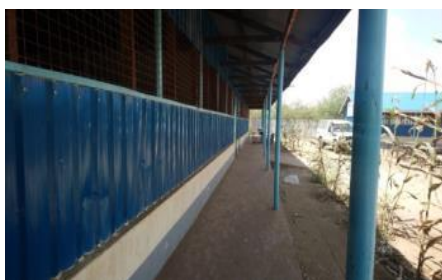
Image 8: A prefab school block
